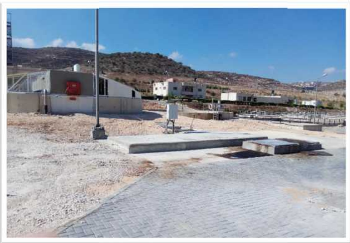
Figure (9): Storage tank of olive mill wastewater
