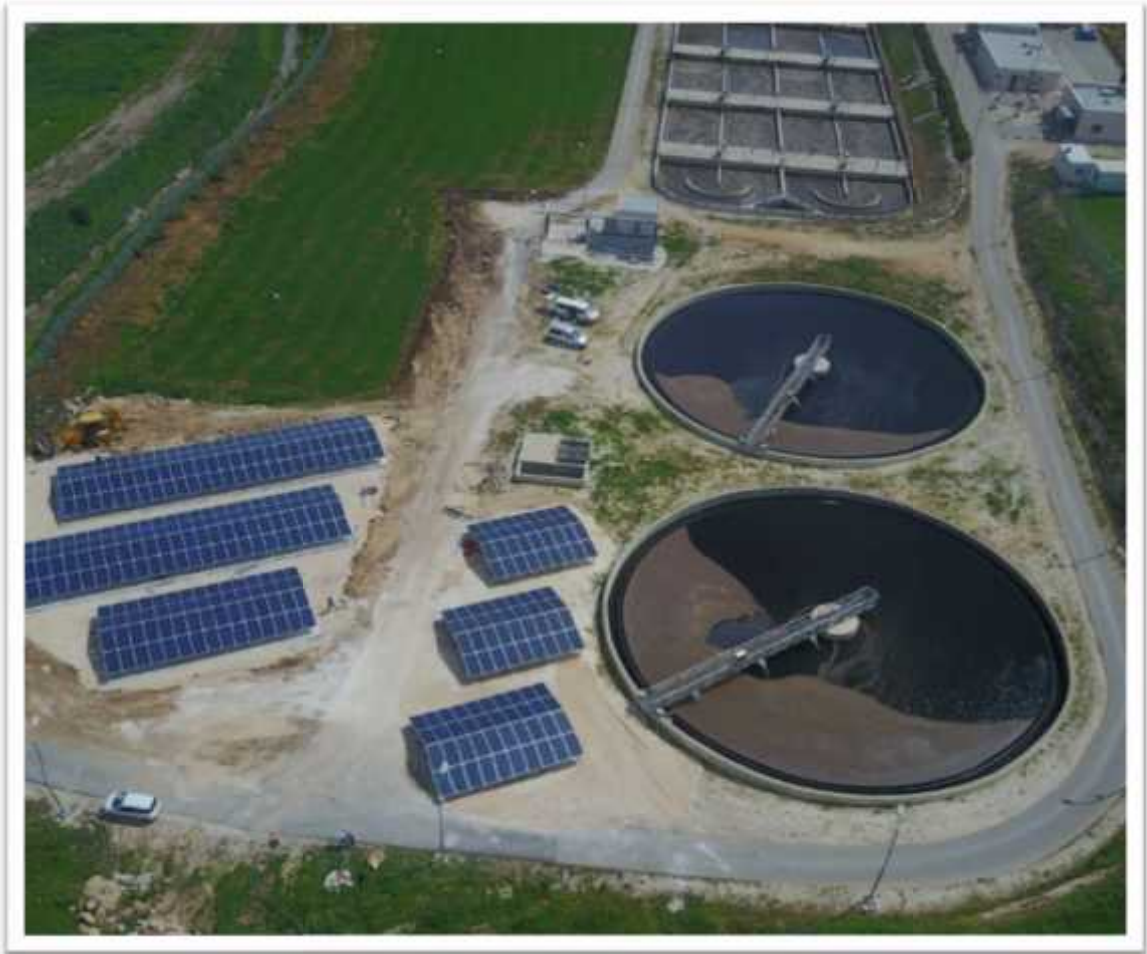
Figure (23): photovoltaic system
