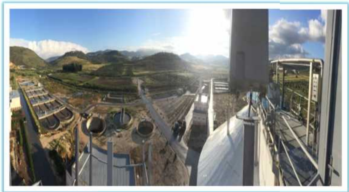
Figure (3): Overview of WWTP Nablus West
