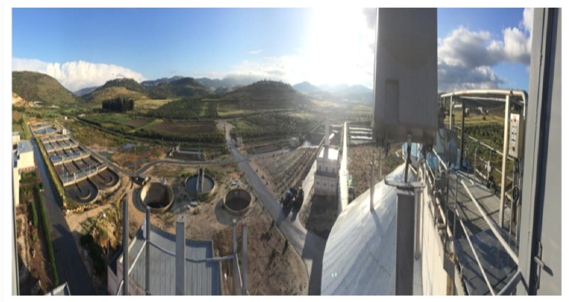
Figure (3): Overview of WWTP Nablus West
