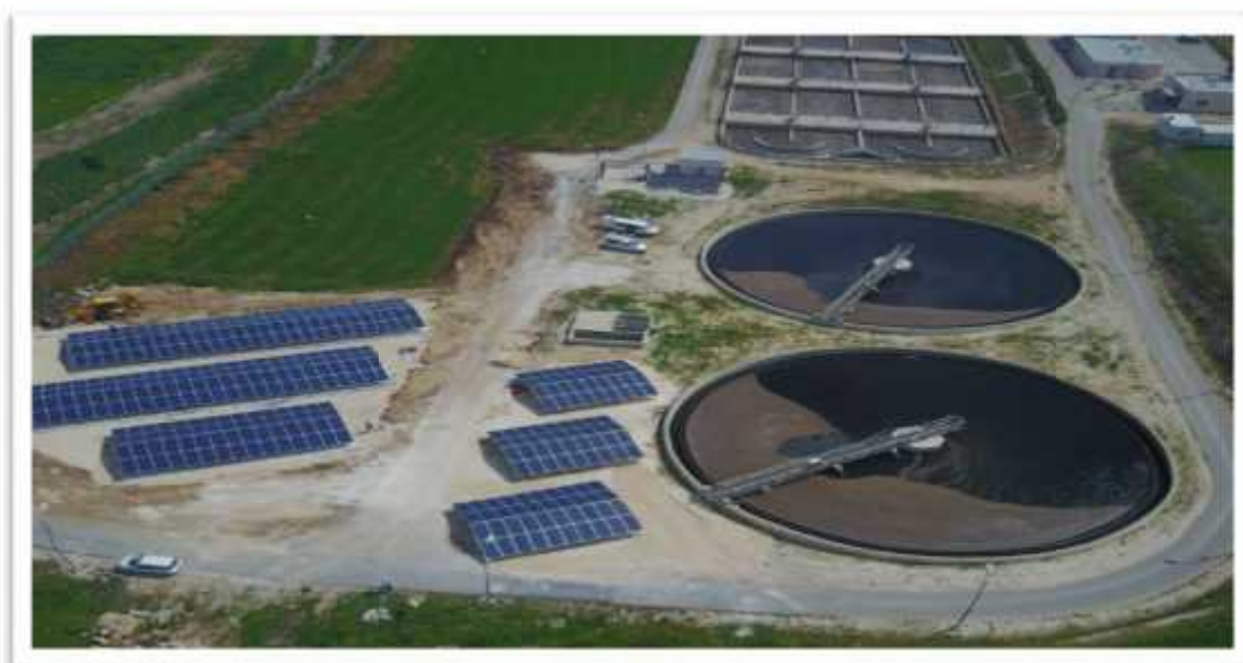
Figure (24): photovoltaic system
