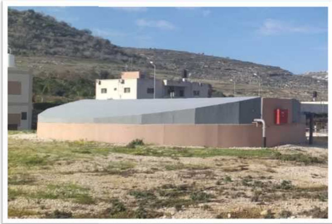
Figure (11): Covering of the primary thickener tank
