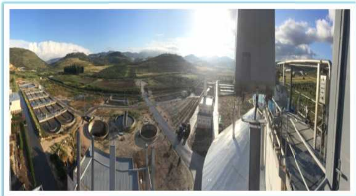
Figure (3): Overview of WWTP Nablus West
