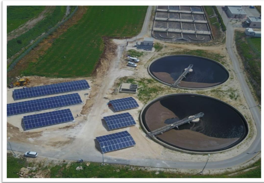
Figure (24): photovoltaic system
