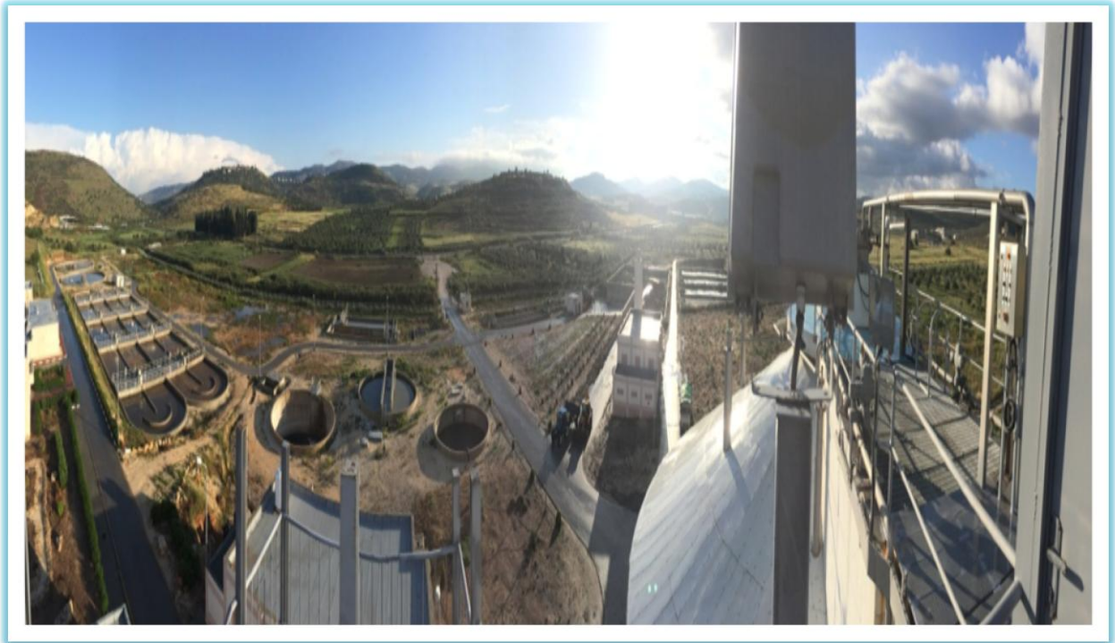
Figure (3): Overview of WWTP Nablus West
