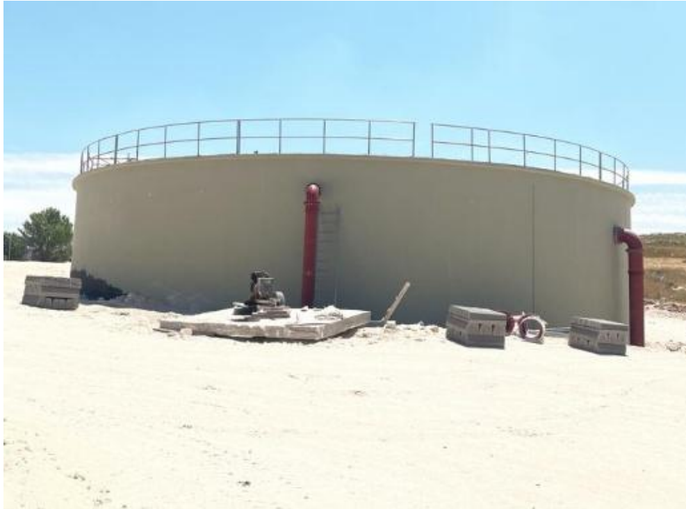
Figure (6): Irrigation reservoir reuse project 2000+
