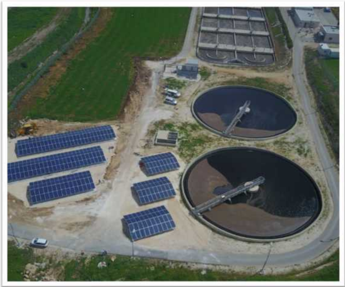
Figure (23): photovoltaic system
