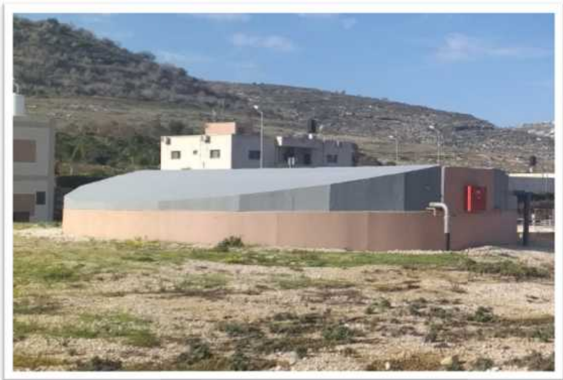
Figure (11): Covering of the primary thickener tank
