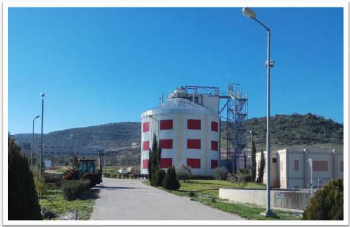
Figure (12): Cladding Rehabilitation of Anaerobic digester roof insulation.
