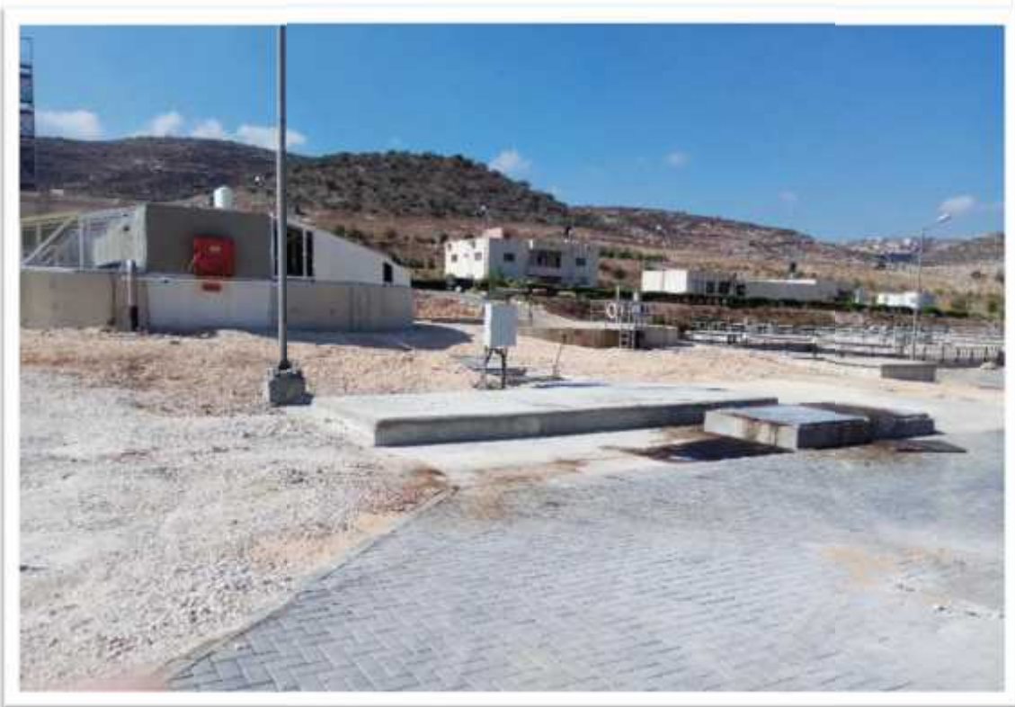
Figure (9): Storage tank of olive mill wastewater
