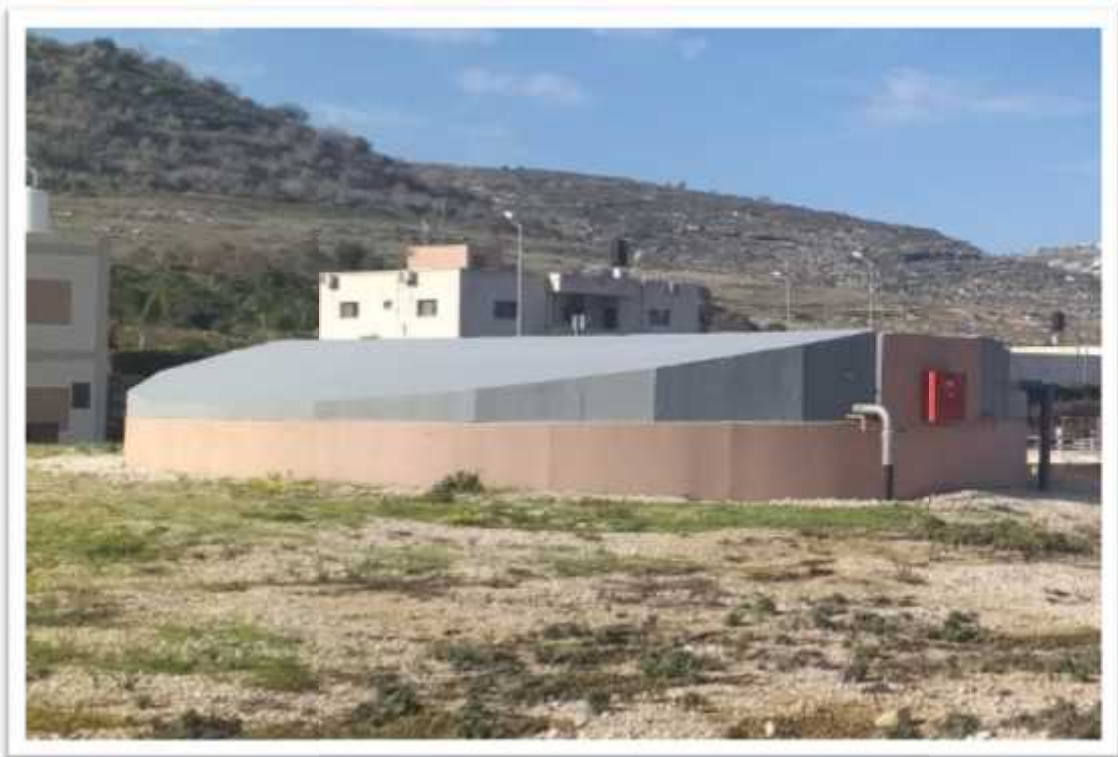
Figure (11): Covering of the primary thickener tank
