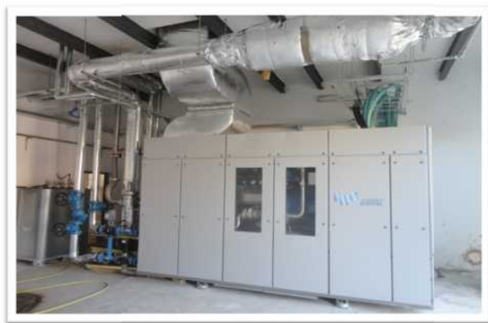
Figure (22): Nablus West CHP engine.
