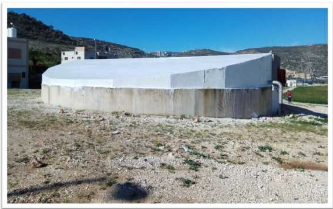
Figure (11): Covering of the primary thickener tank
