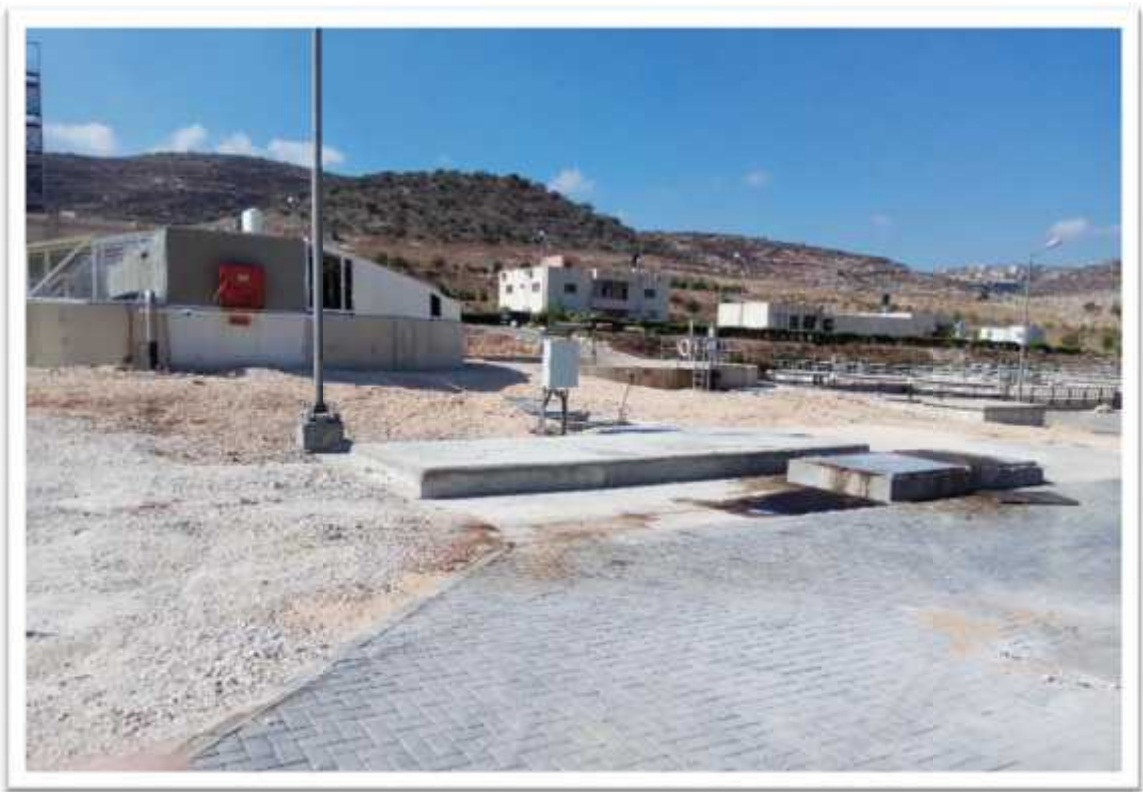
Figure (9): Storage tank of olive mill wastewater
